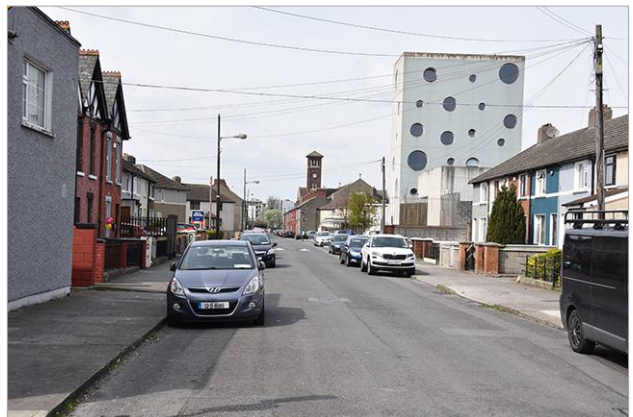
Plate 13.12: View west from St. Mary's Road
